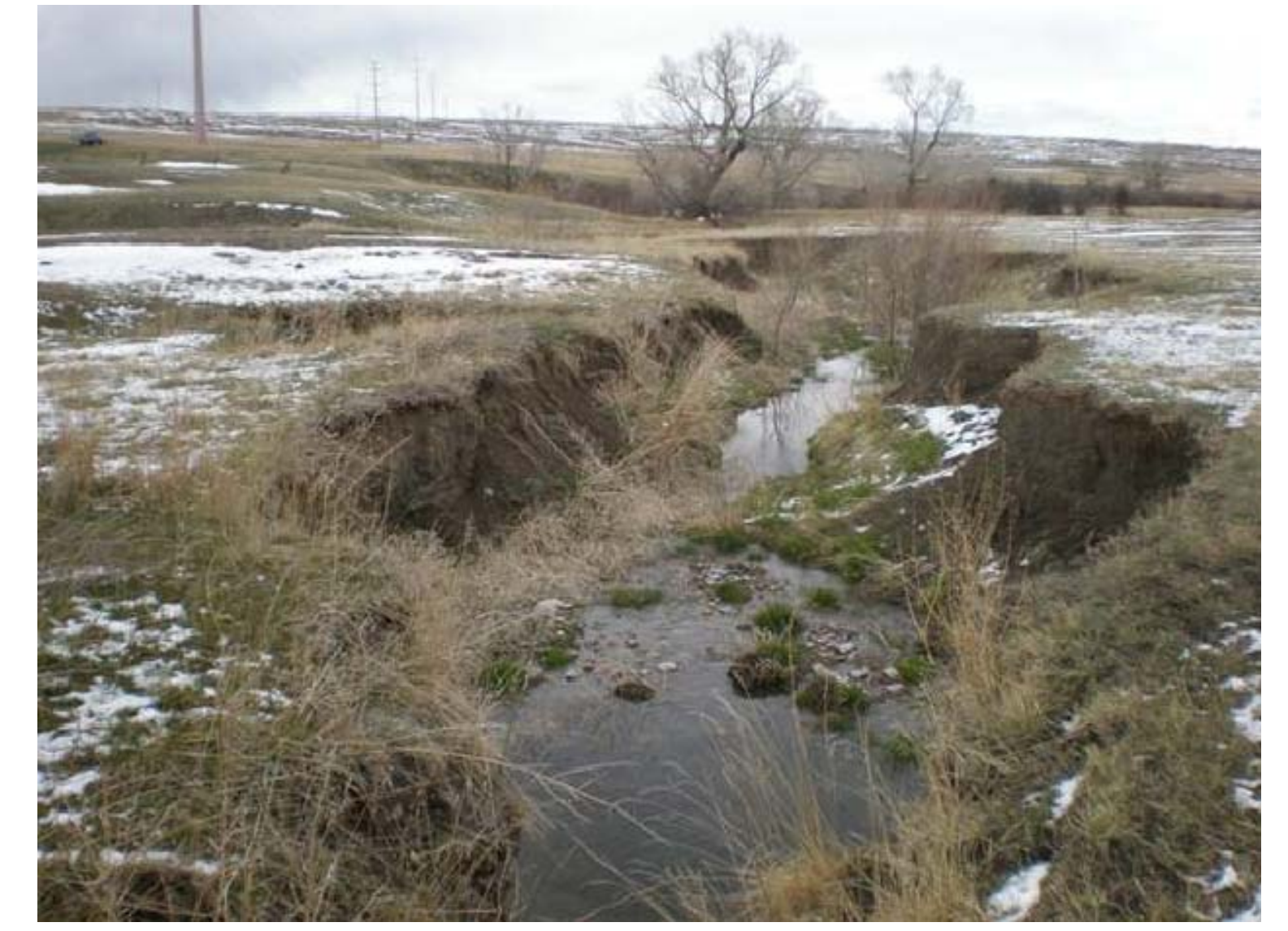
BEFORE NATURAL CHANNEL CONSTRUCTION
