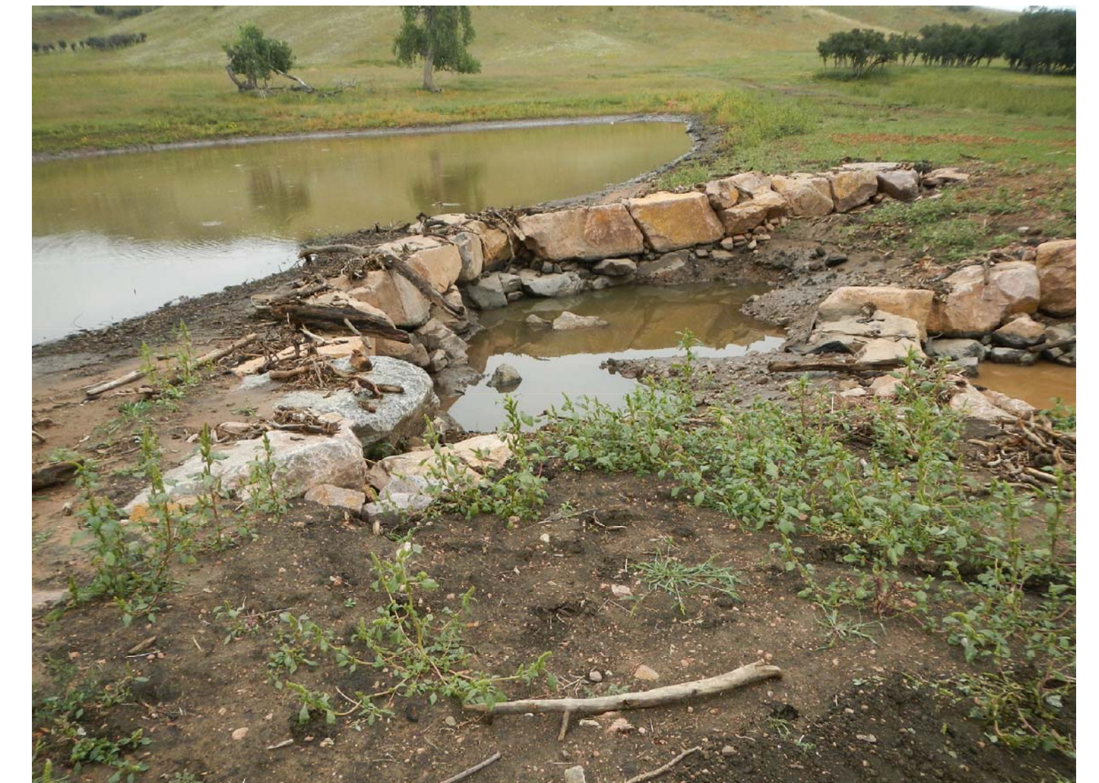
CONSTRUCTED ROCK VANE
